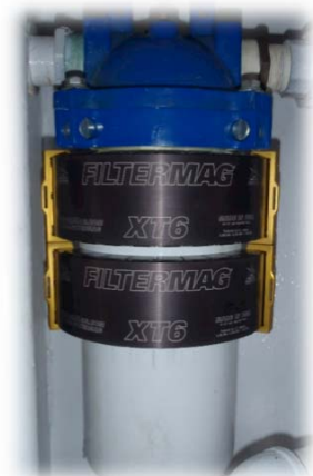
FilterMag on the outside . . . placement of XT6s on bulk fuel filter.
