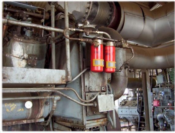
Two CT4.9s installed on turbo oil filters (5.5 inch diameter).
